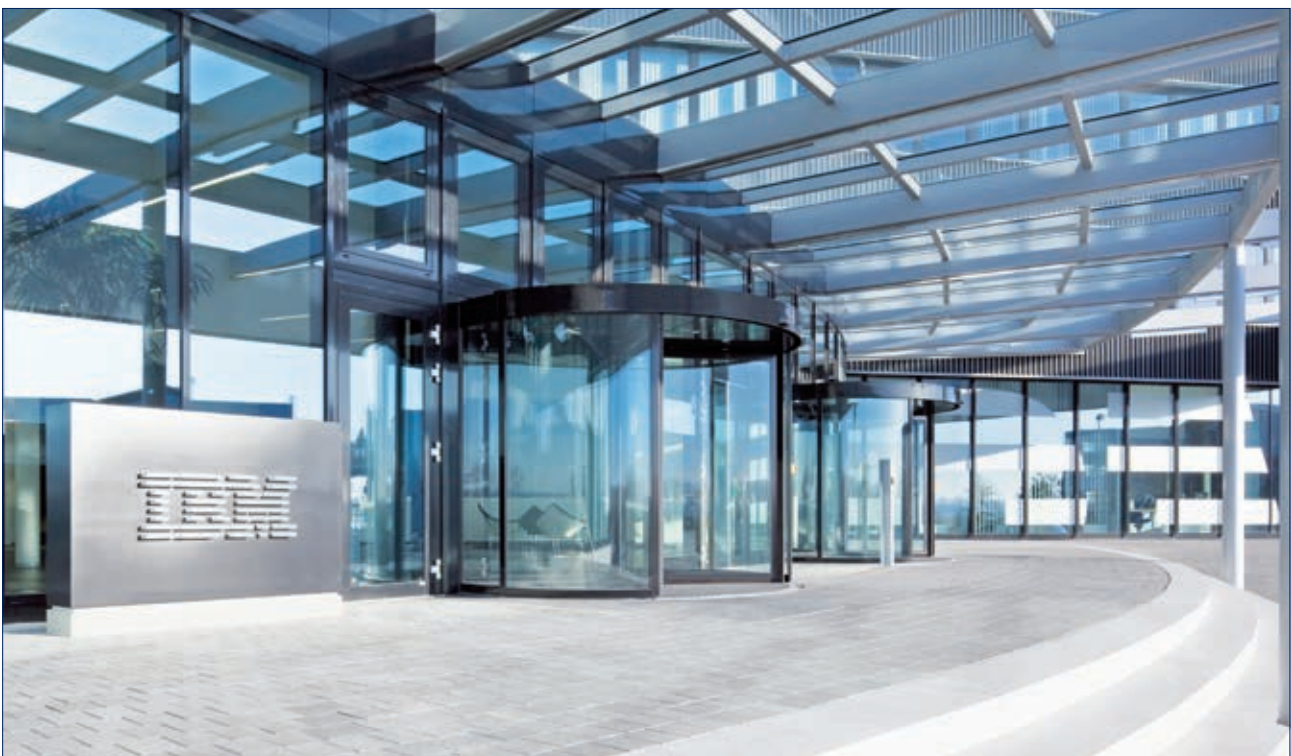
IBM Ehningen, Germany (Photo: GEZE GmbH)
