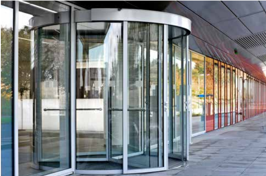
Hitachi Power, Duisburg, Germany (photo: Lothar Wels / GEZE GmbH)
