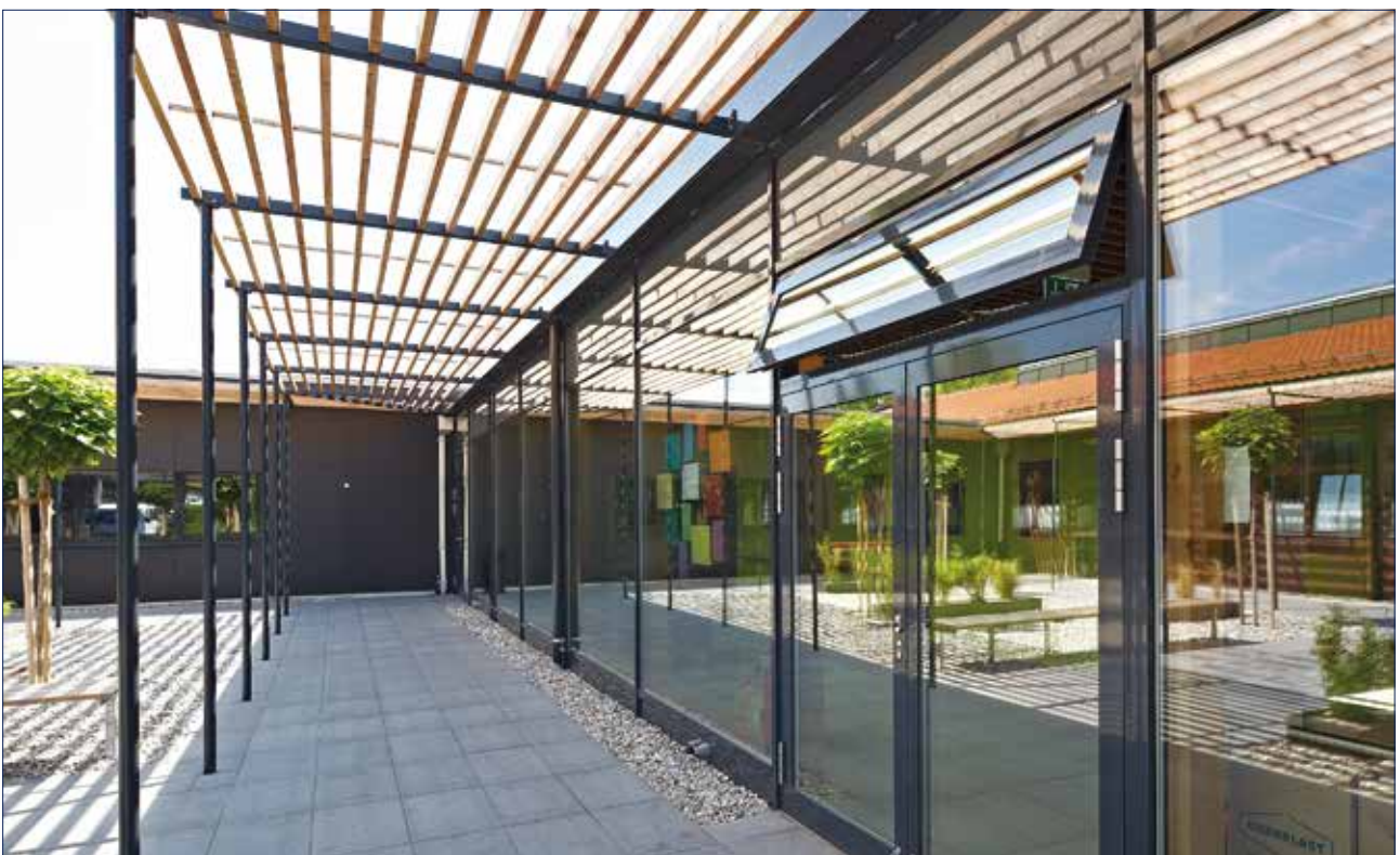
Ecksberg Foundation, Mühlendorf, Germany (Photo: Robert Sprang)
